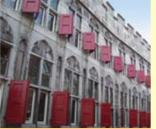
Donkerstraat 15-19. The façade of this property is built of Namur stone, a grey, fine-grained limestone from the Lower Carboniferous that was extracted in the Maas valley near the Belgian city of Namur. The façade was built in the second half of the fifteenth century. The coat of arms in the façade is made of 'mergel', a fine-grained
